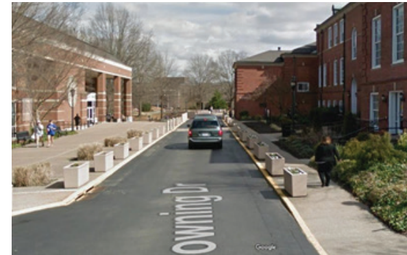
Existing Browning Street
